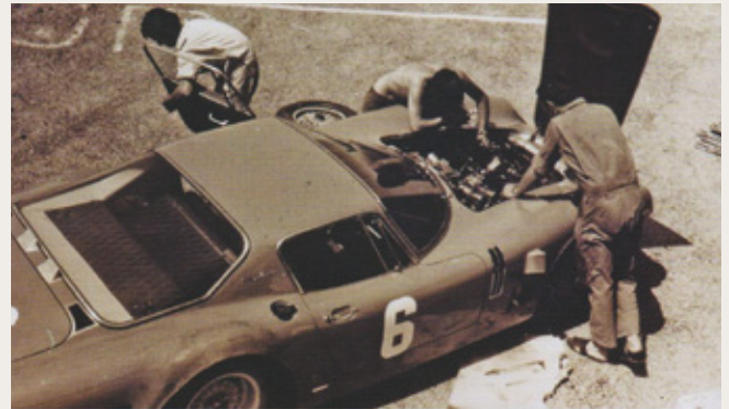
23/07/1967 - Coppa Emilio Materazzi, Mugello 500kms road race, mechanics working on the car in heat (44 C°), Weber set up and recent wheel-arch extension are clearly visible ©DR
